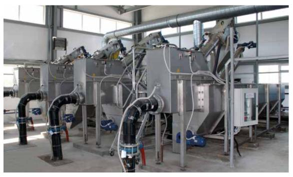
Each compact pre-treatment plant has a capacity of up to 30 litres per second and offers the operator optimum efficiency in mechanical pre-treatment and grit separation, which greatly benefits the subsequent biological and chemical treatment steps of the effluent in its purification process.
